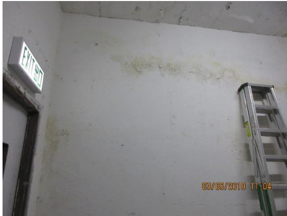
Internal side of external wall
